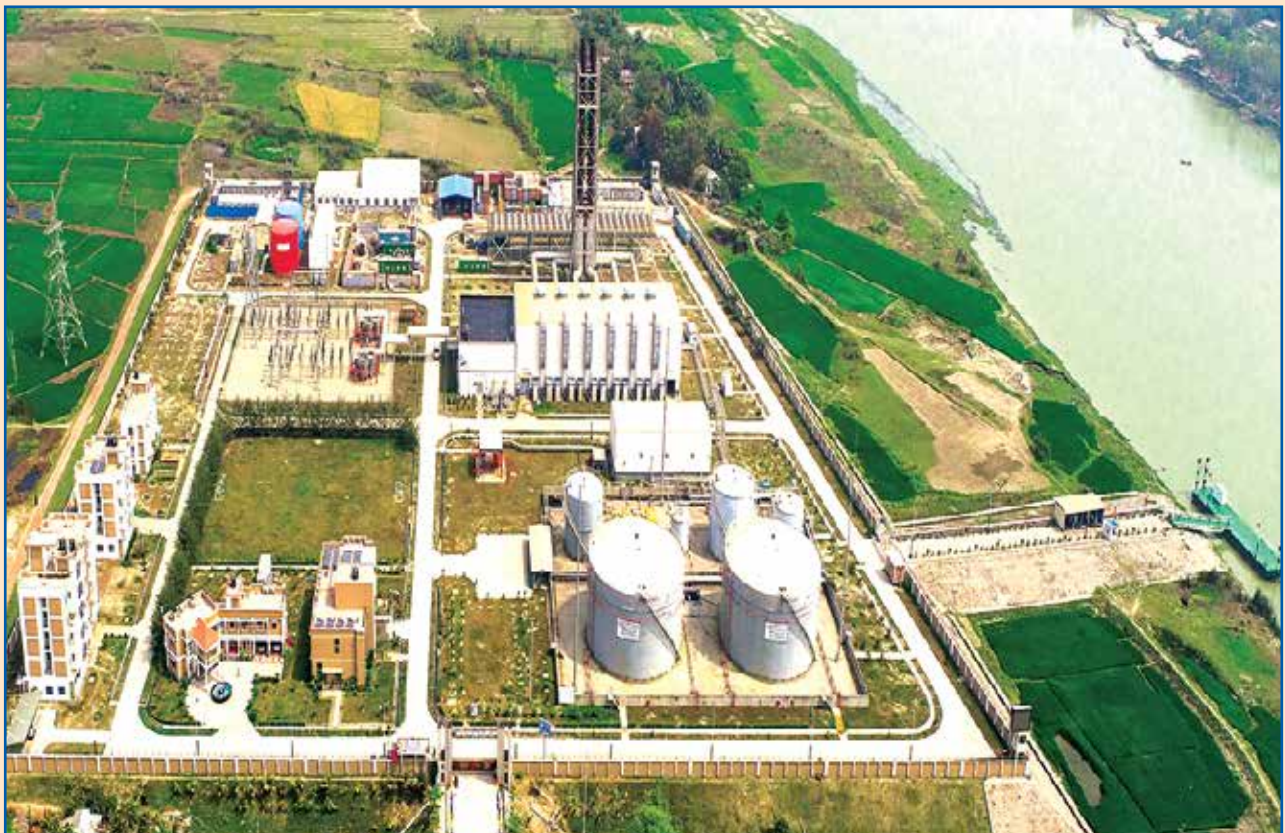
Madhumati 100 MW Power Plant
