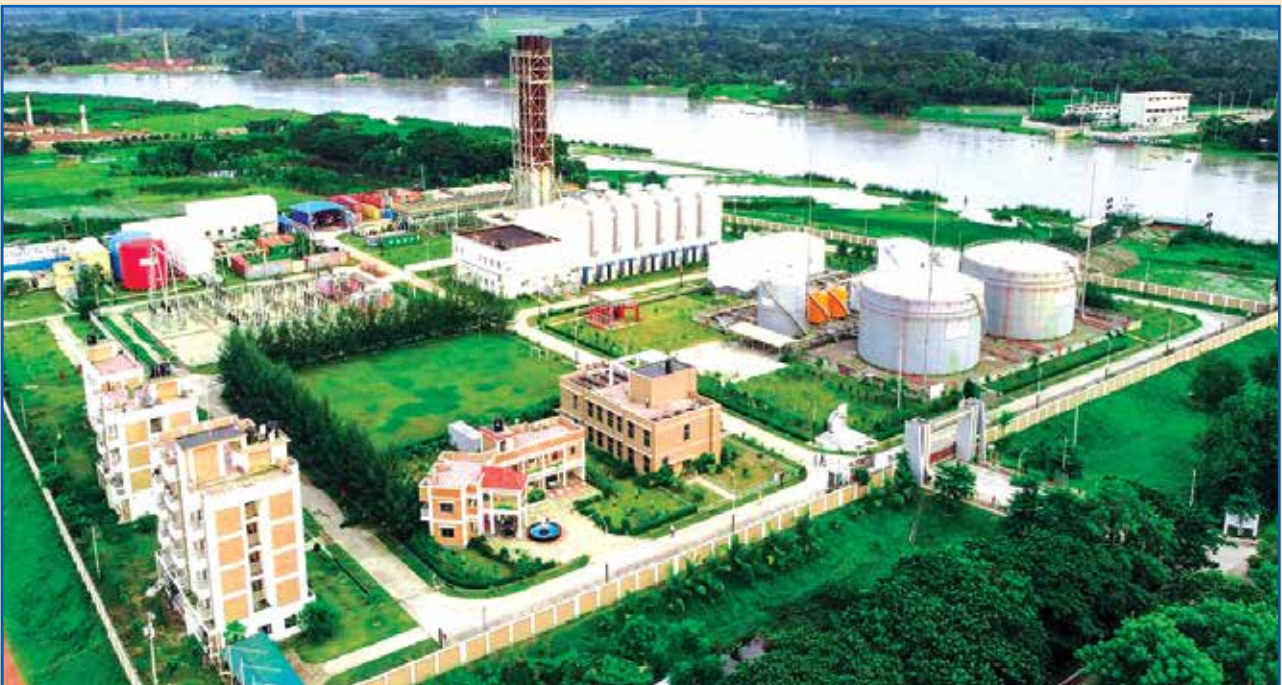
Madhumati 100 MW HFO Based Power Plant
