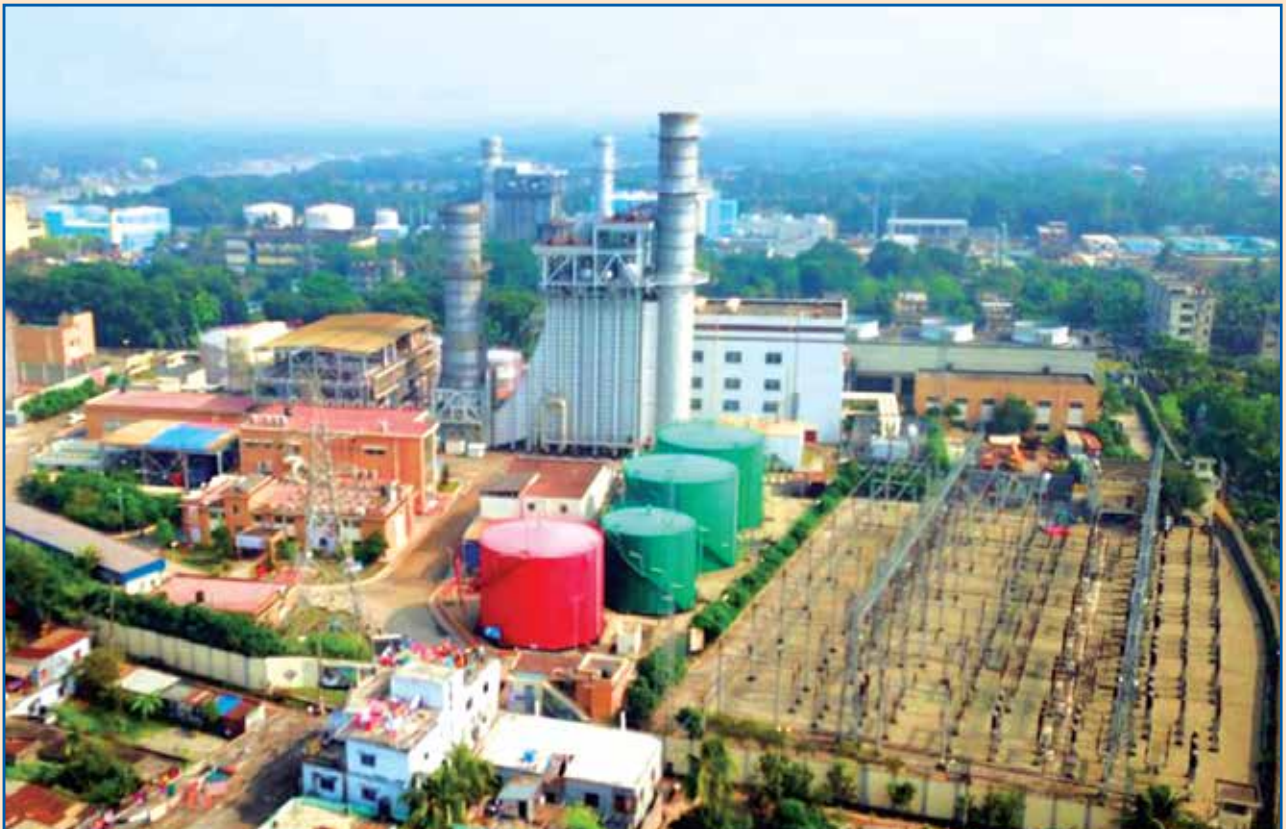
Khulna 225 MW Combined Cycle Power Plant
