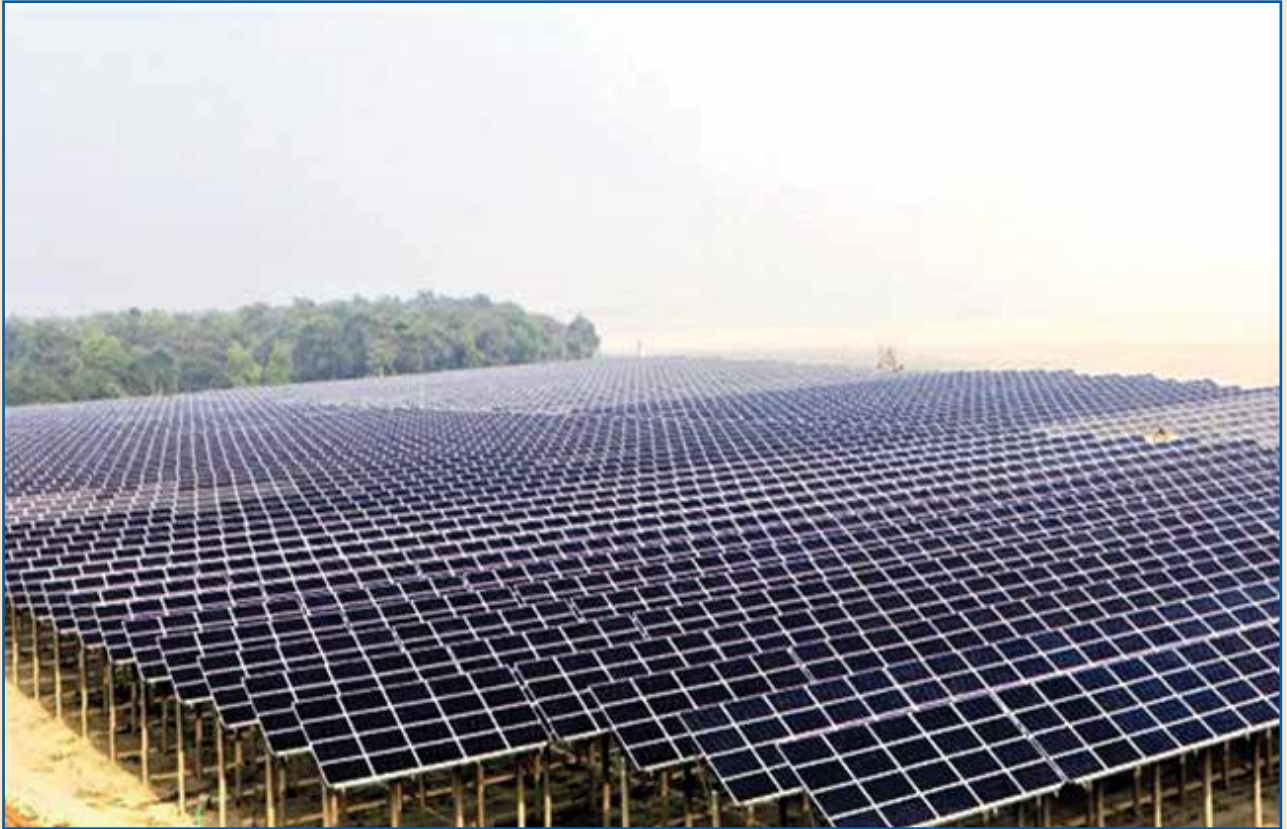
Sirajganj 7.6 MWp Grid Connected Photovoltaic Solar Power Plant
