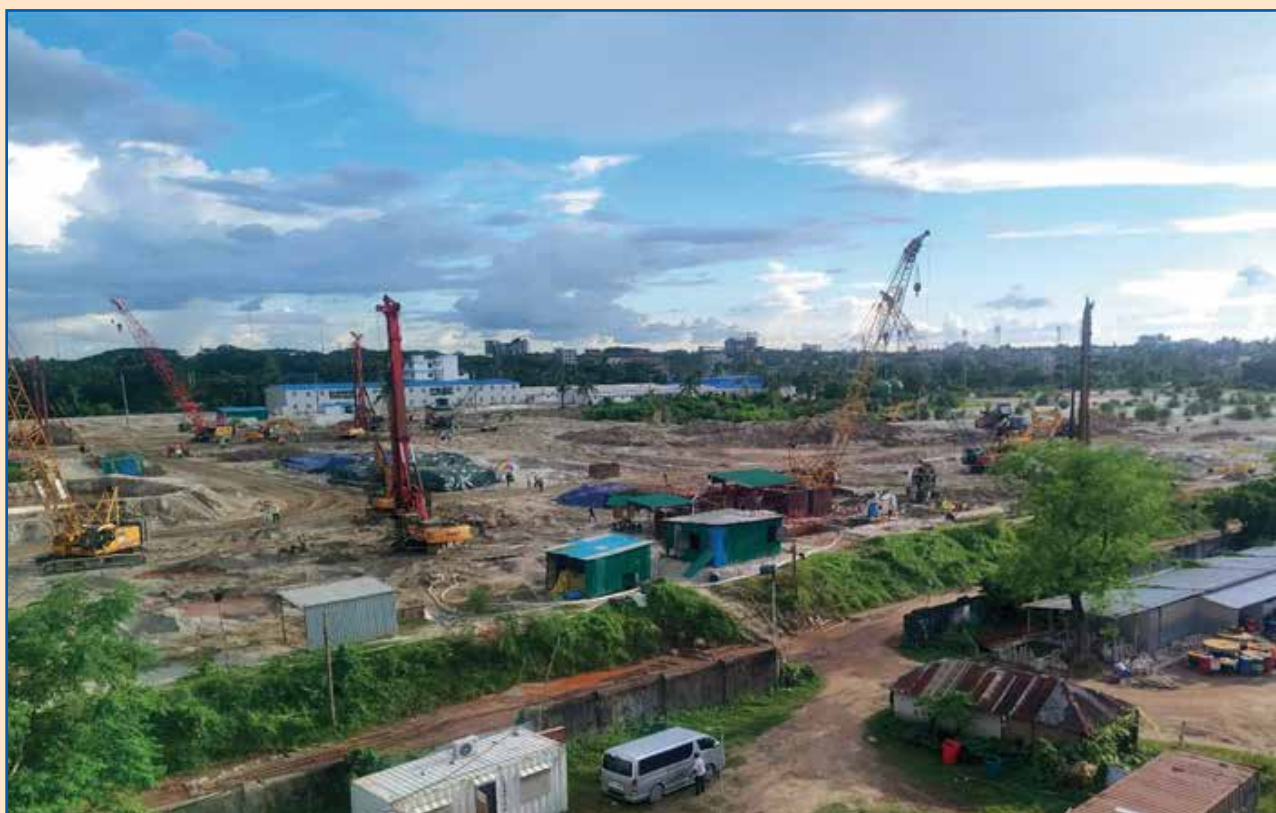
Rupsha 800 MW Combined Cycle Power Plant Project Site
