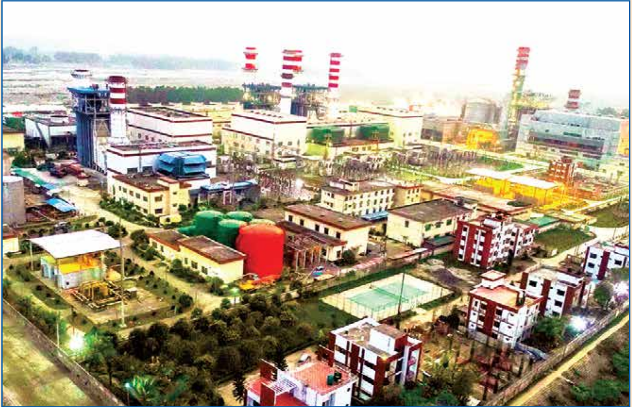
Sirajganj Power Generation Hub (Unit:1, 2, 3 & 4)
