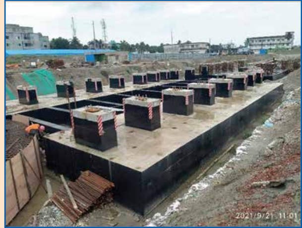
HRSG-1 area at Rupsha 800 MW Combined Cycle Power Plant Project Site
