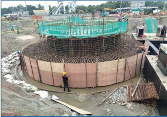
Main Stack-1 Foundation area at Rupsha 800 MW Combined Cycle Power Plant Project Site
