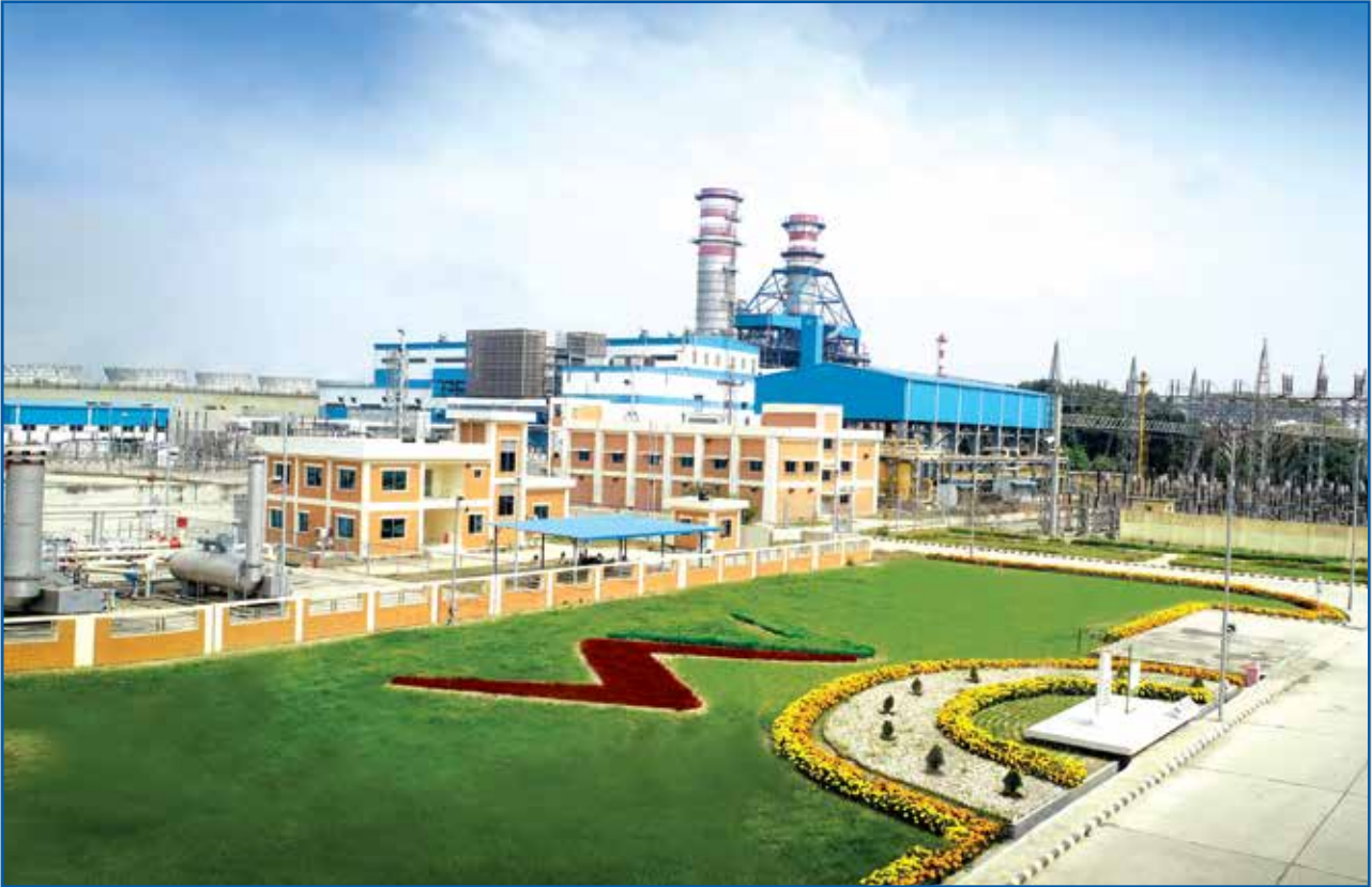
Bheramara 410 MW Combined Cycle Power Plant
