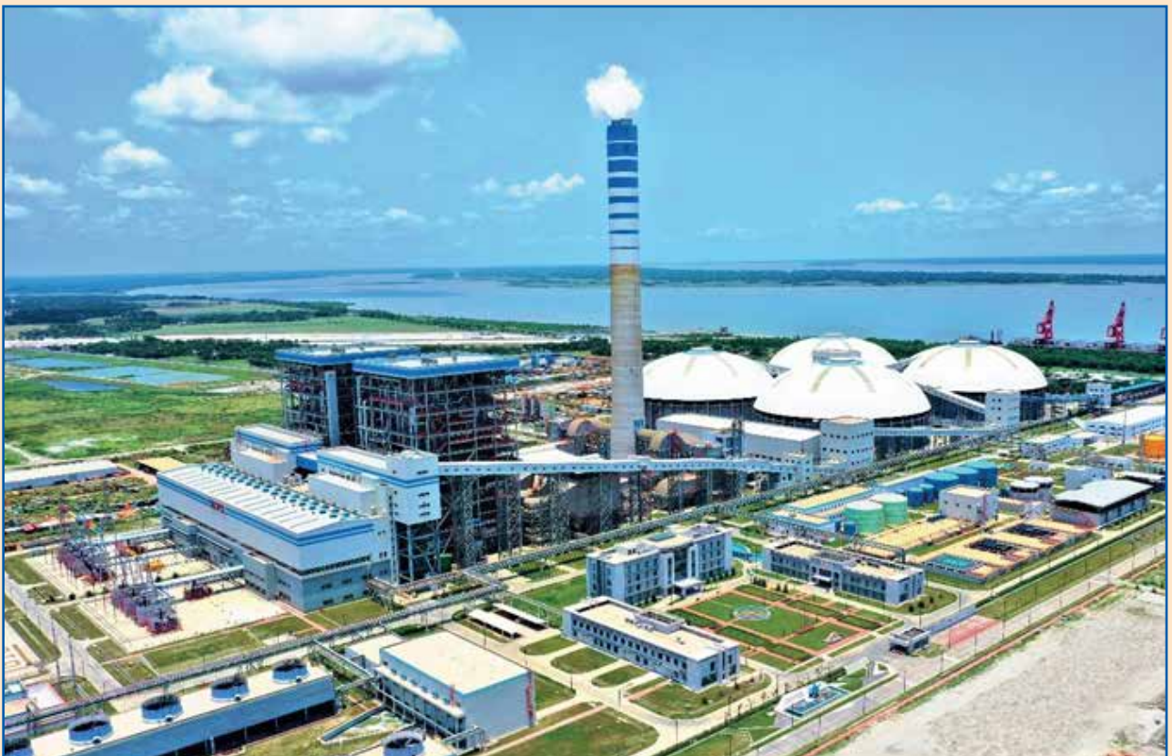
Payra 1320 MW Thermal Power Plant (1st Phase) (Under JVC)
