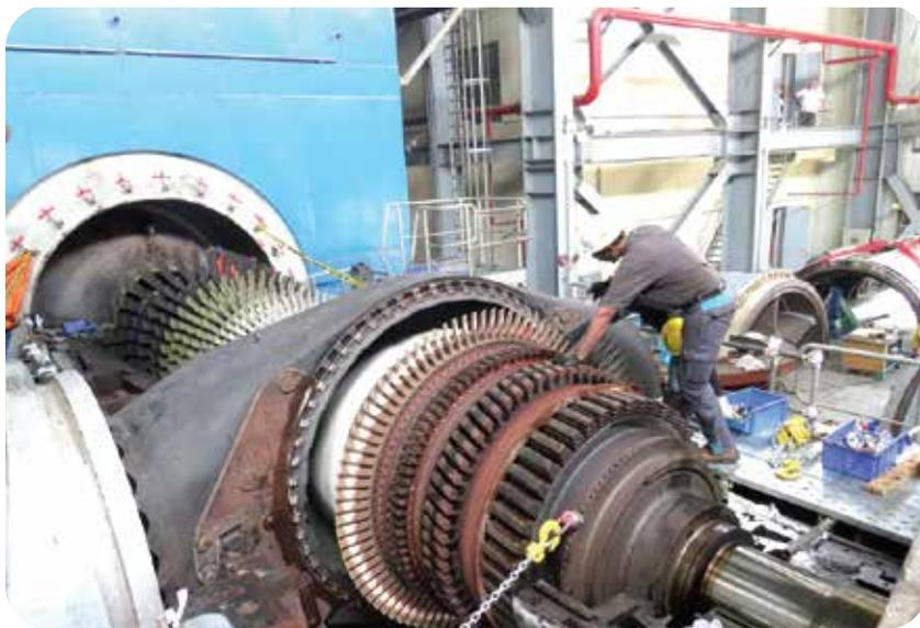
Removing of Turbine's Old Blades during HGPI Work at Sirajganj 225 MW CCPP
