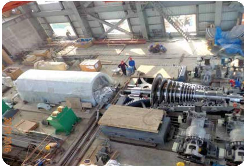
Erection of Generator & Turbine of Upgradation of Khulna 150 MW to 225 MW CCPP Project
