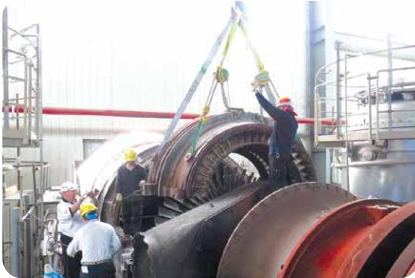
Removing of Turbine's Upper Casing during HGPI Work at Sirajganj 225 MW CCPP
