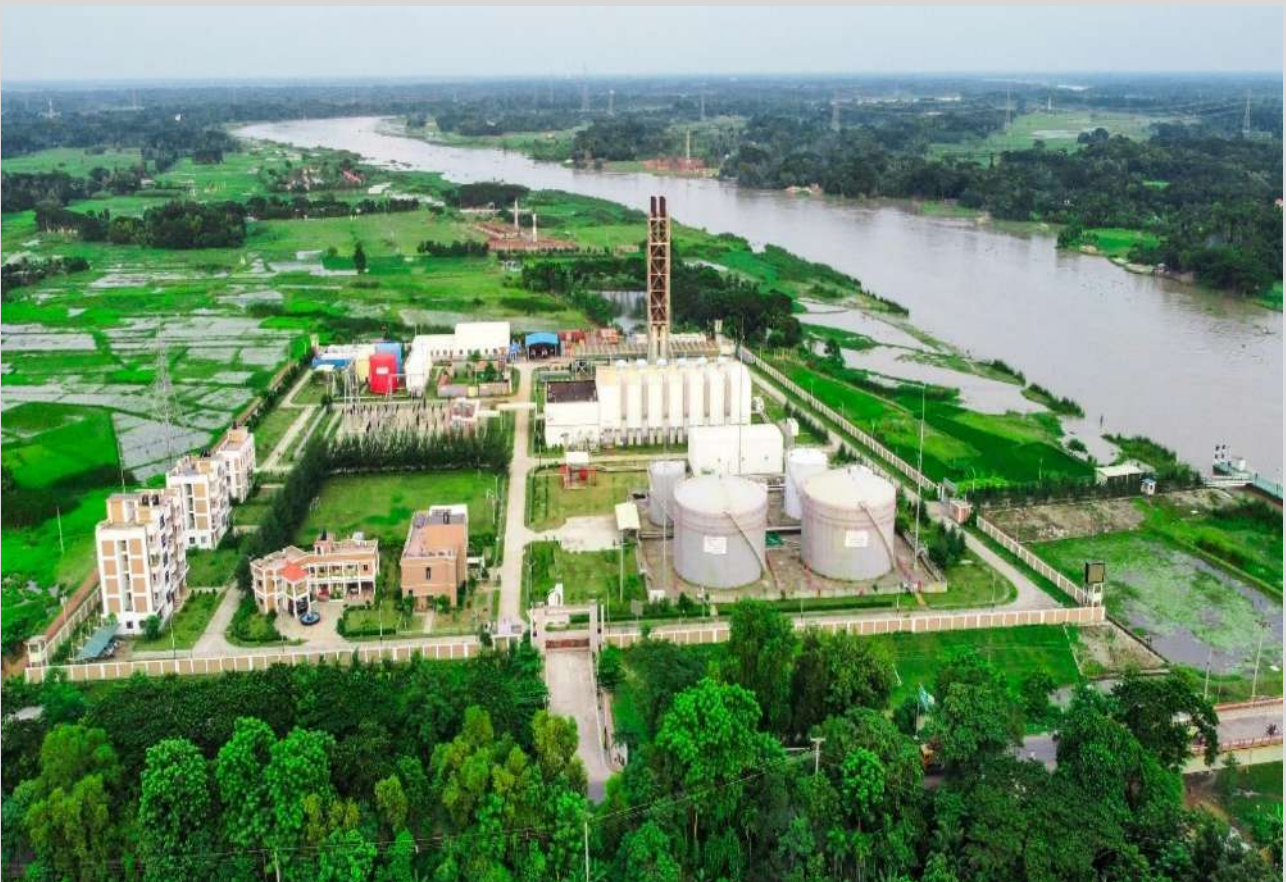
Madhumati 100 MW Power Plant
