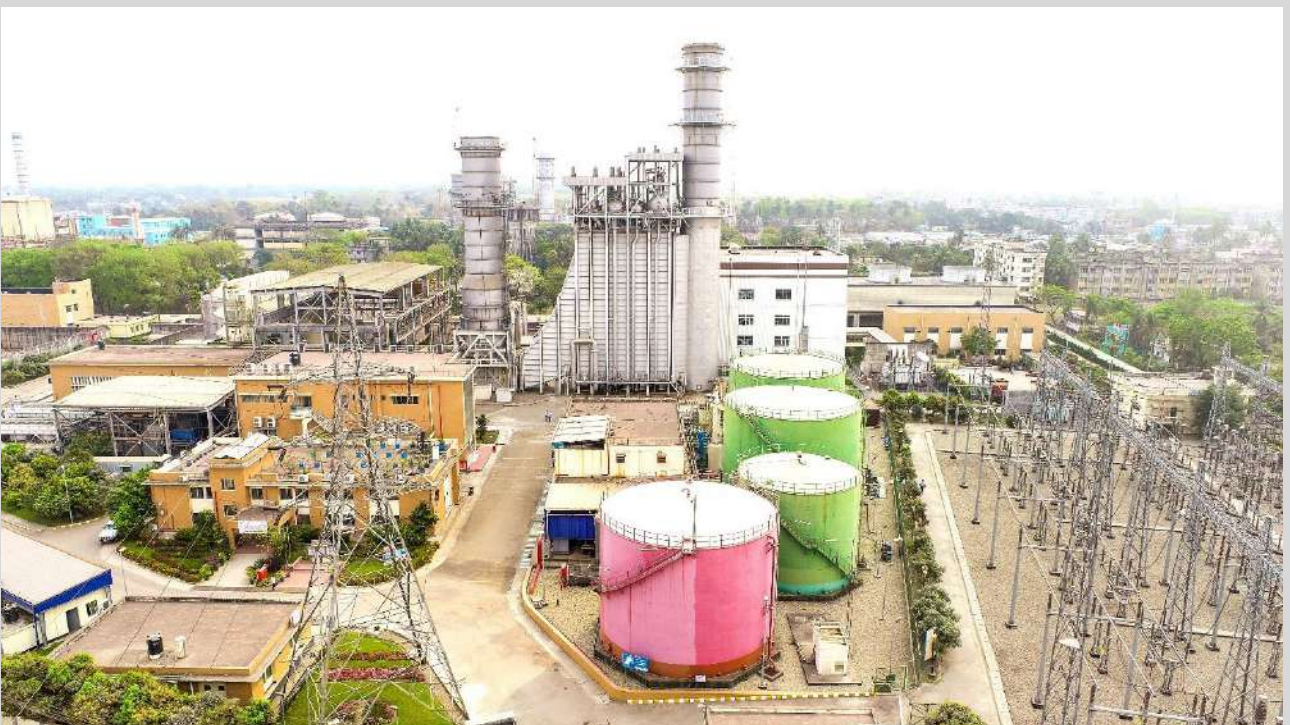
Khulna 225 MW Combined Cycle Power Plant
