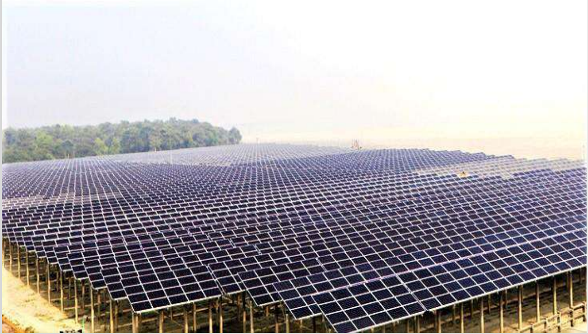
Sirajganj 7.6 MWp Grid Connected Photovoltaic Solar Power Plant
