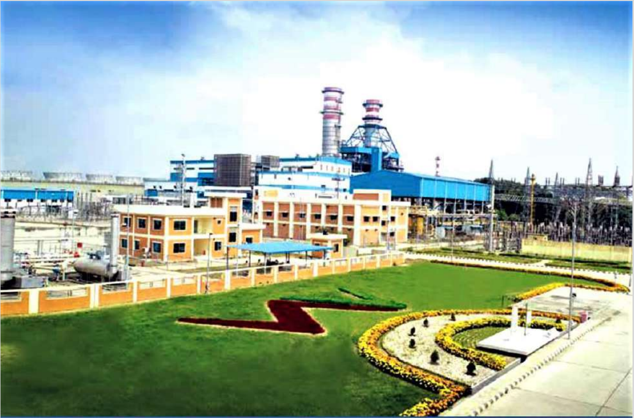
Bheramara 410 MW Combined Cycle Power Plant
