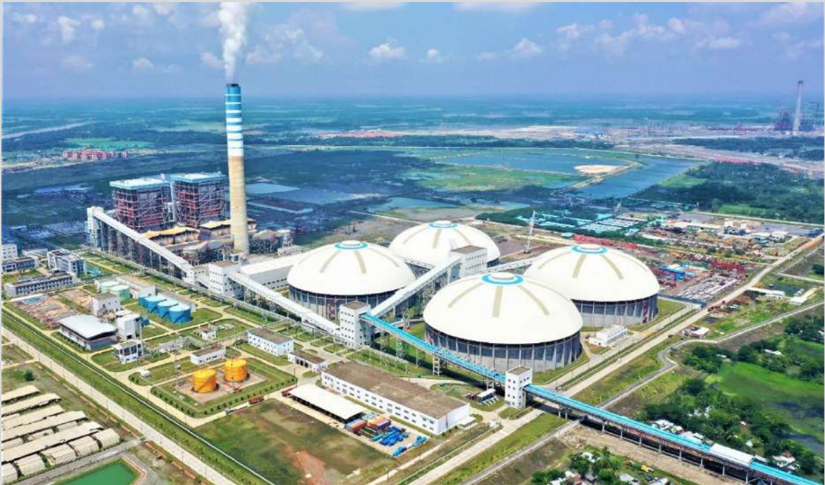
Payra 1320 MW Thermal Power Plant (1 st Phase) (Under JVC)
