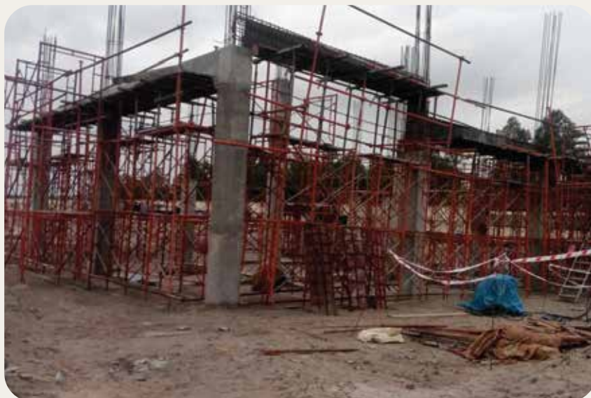
GIS Control Building- Sirajganj 400 MW ( \pm 10\% ) Combined Cycle Power Plant Project
