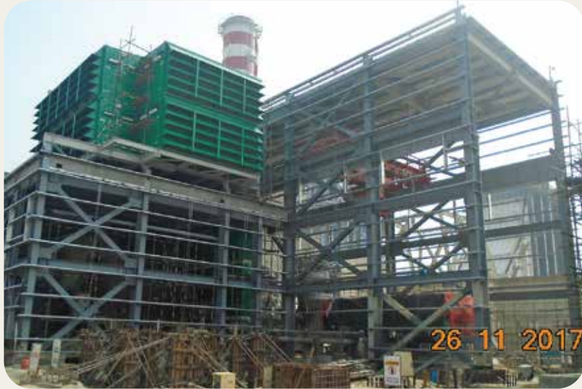
GTG Building- Sirajganj 225 MW CC Power Plant Project (3rd Unit)
