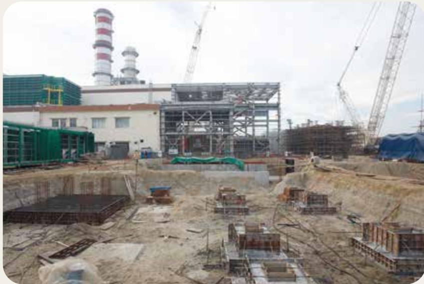
EPC Work of Sirajganj 225 MW CC Power Plant Project (3rd Unit)
