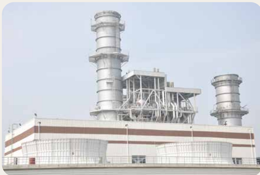
Khulna 225 MW CC Power Plant
