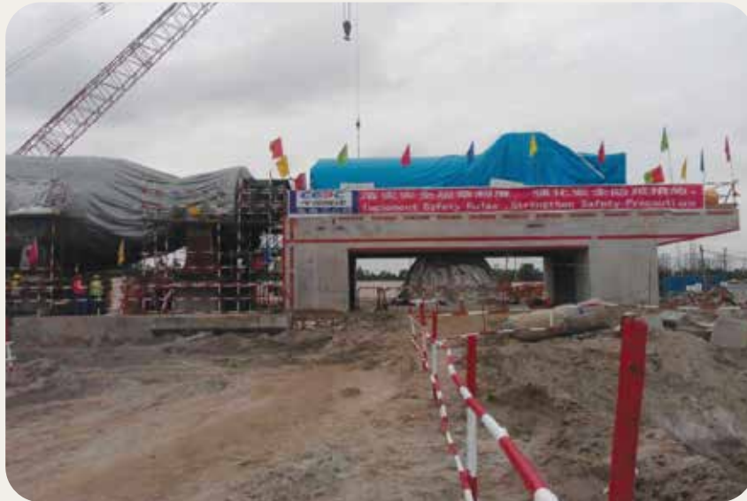
GT & GTG- Sirajganj 400 MW ( \pm 10\% ) Combined Cycle Power Plant Project
