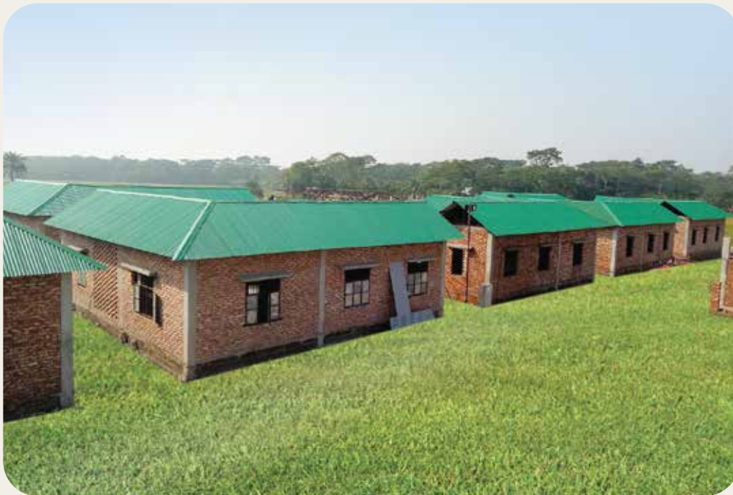
Rehabilitation at Payra 1320 MW TPP Project site
