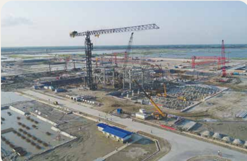
Aerial View of EPC Work of Payra 1320 MW Thermal Power Plant Project
