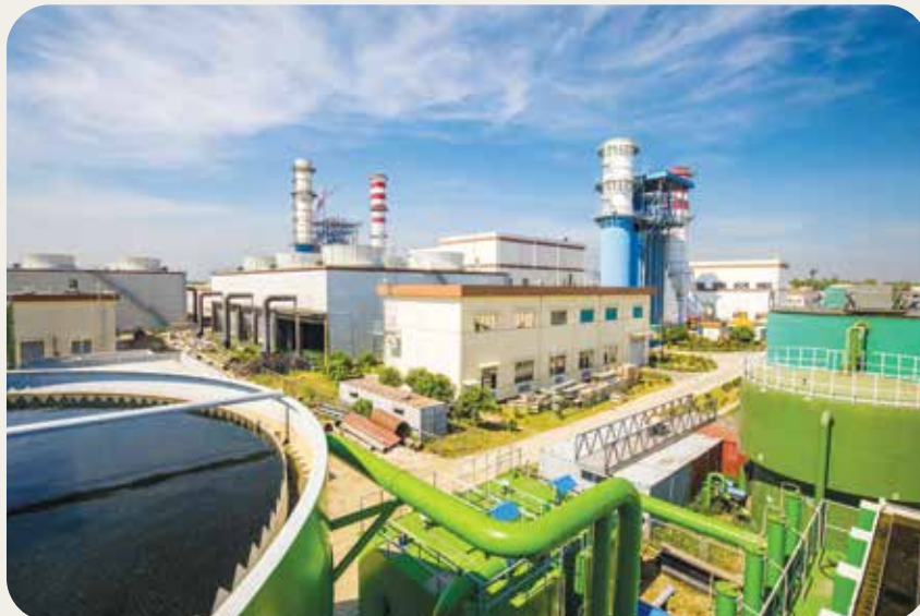
Sirajganj 225 MW CC Power Plant (1st & 2nd Unit)
