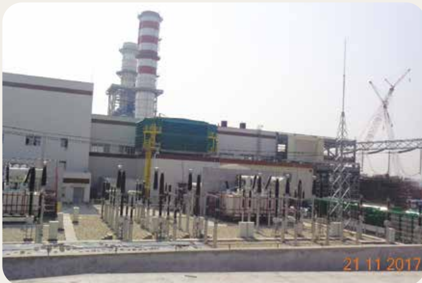
EPC Work of Sirajganj 225 MW CC Power Plant Project (2nd Unit)
