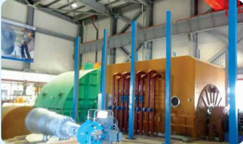
Steam Turbine & ST Generator at Sirajganj 225 MW CCPP Project (Unit-3)
