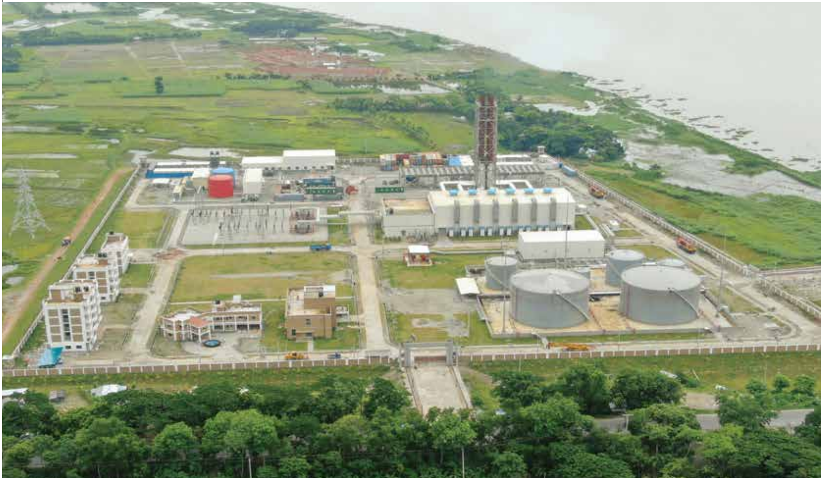
Madhumati 100 MW HFO Based Power Plant
