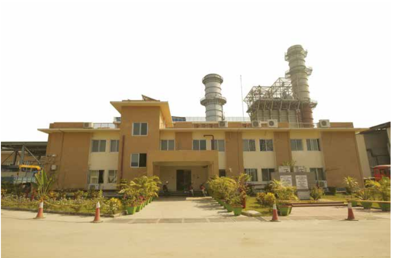
Khulna 225MW Combined Cycle Power Plant
