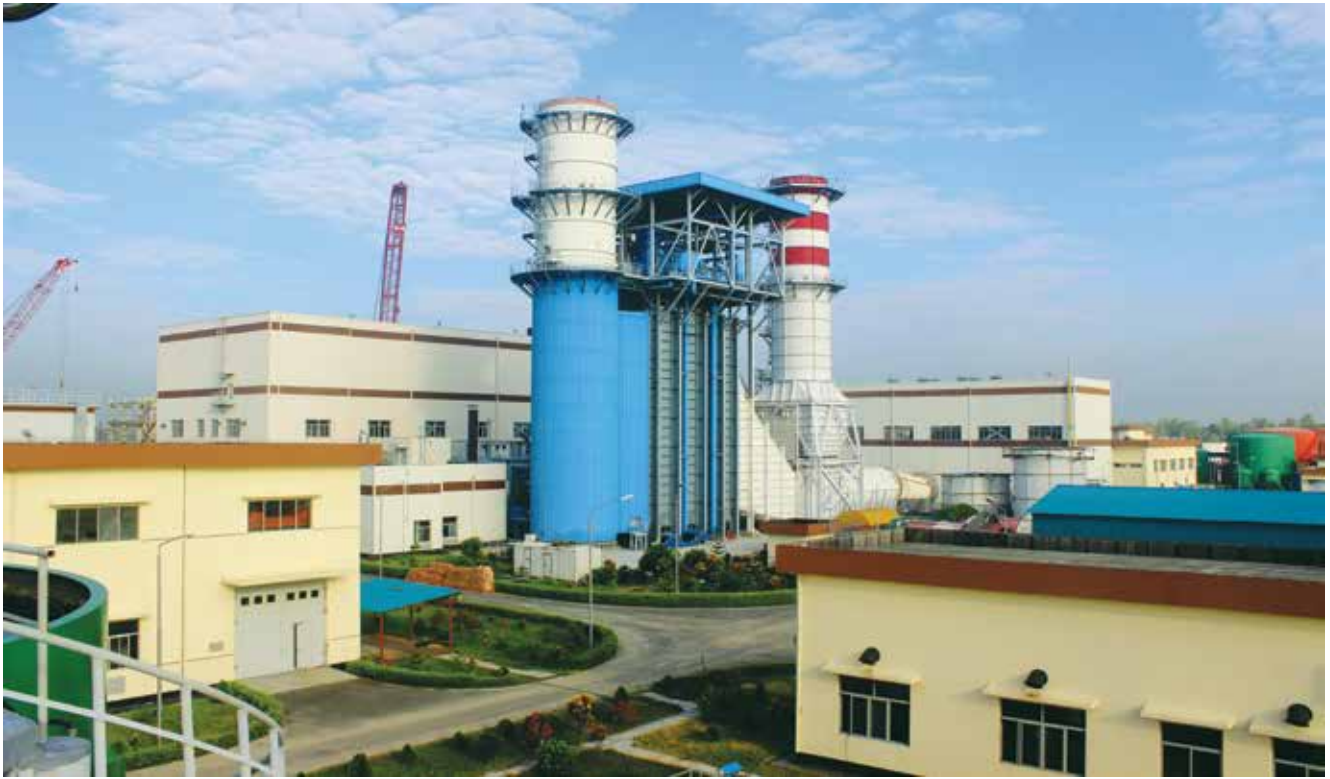
Sirajganj 225 MW Combined Cycle Power Plant (Unit-1)
