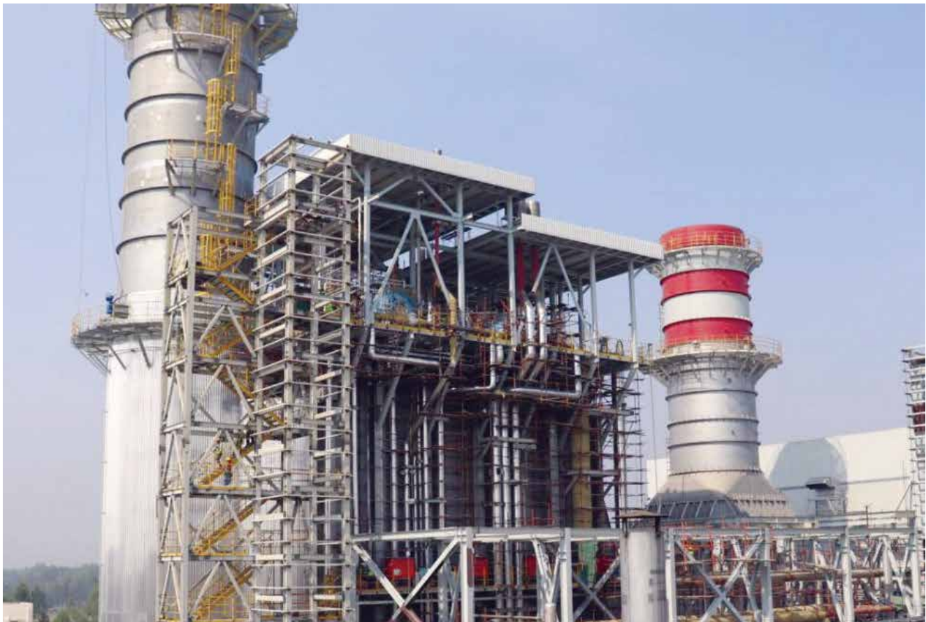
Sirajganj 414 MW Combined Cycle Power Plant (Unit-4) (Under JVC)
