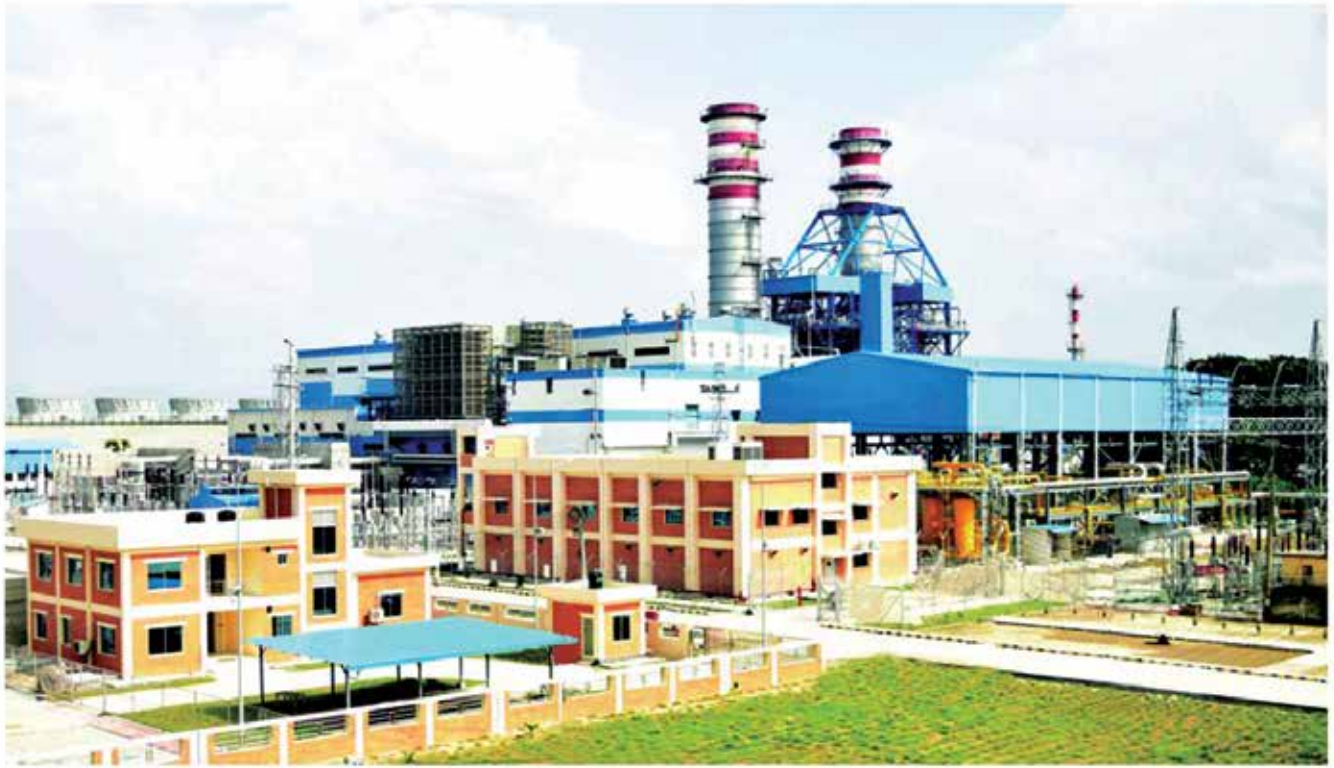
Bheramara 410 MW Combined Cycle Power Plant
