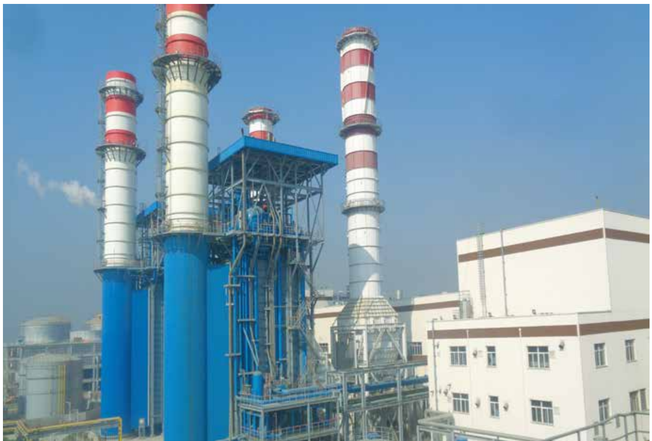
Sirajganj 225 MW Combined Cycle Power Plant (Unit-2)
