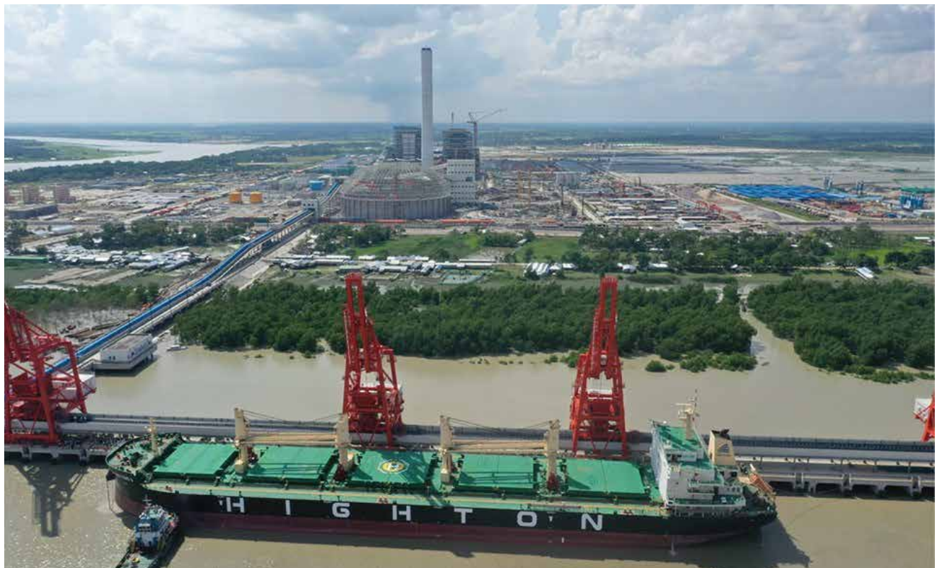
First Arrival of Coal at Payra 1320 MW Thermal Power Plant (1st Phase) (Under JVC)
