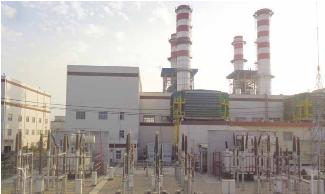
Sirajganj 225 MW Combined Cycle Power Plant (Unit-3)
