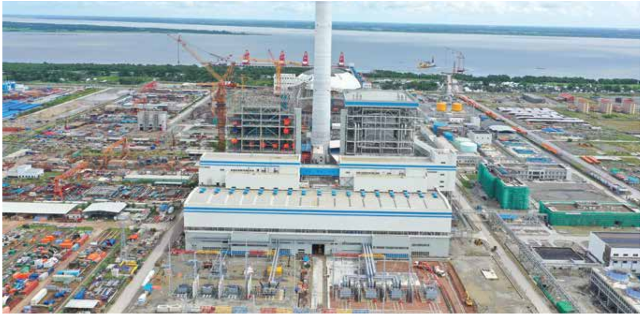
Payra 1320 MW Thermal Power Plant Project (1 st Phase)
