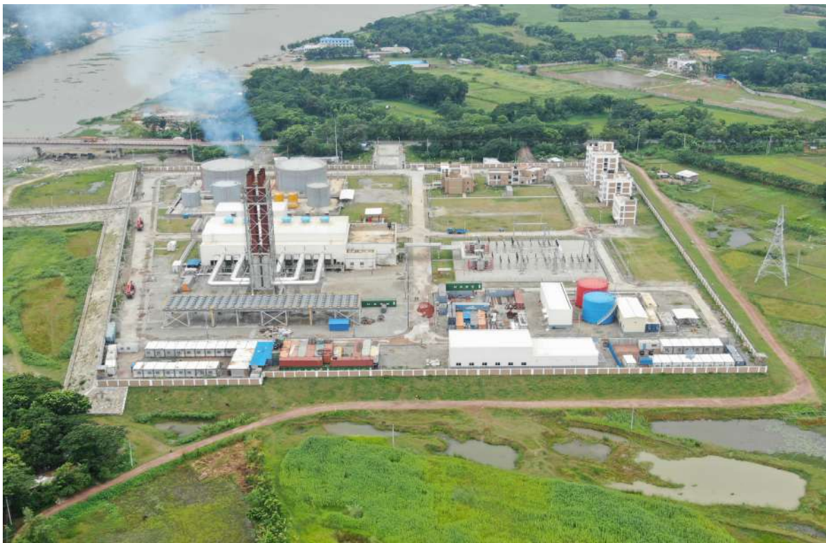
Madhumati 100 MW HFO Based Power Plant
