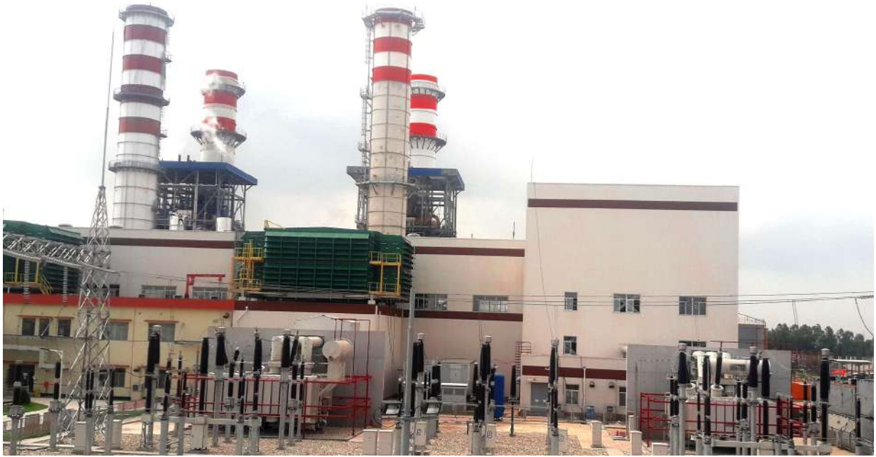
Sirajganj 225 MW Combined Cycle Power Plant (3 rd Unit)
