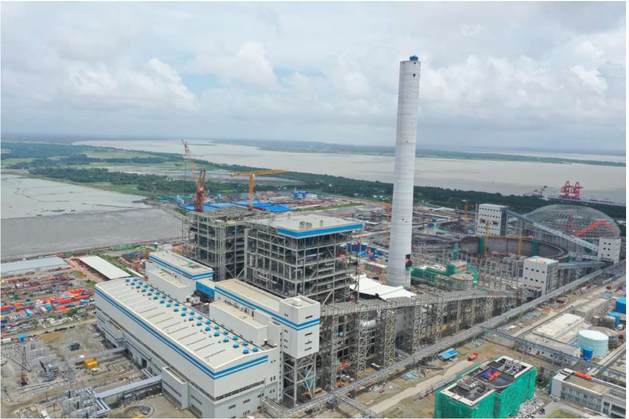
Payra 1320 MW Thermal Power Plant (1 st Phase) (Under JVC)
