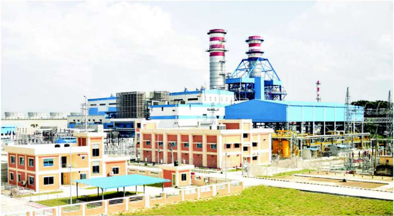
Bheramara 410 MW Combined Cycle Power Plant
