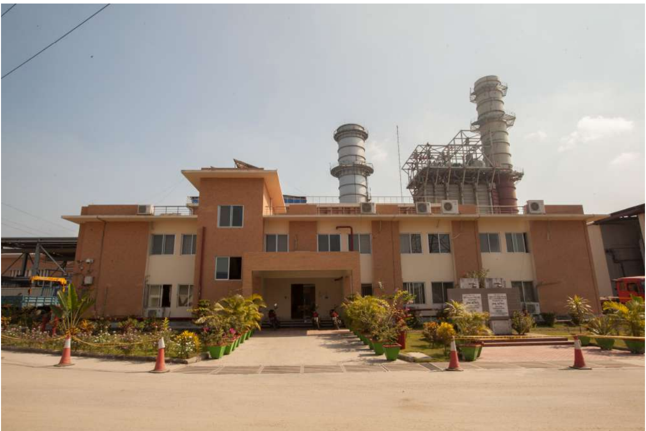
Khulna 225 MW Combined Cycle Power Plant
