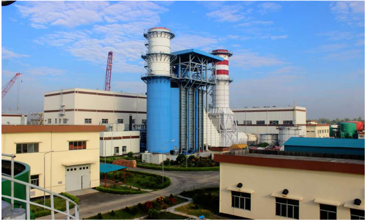
Sirajganj 225 MW Combined Cycle Power Plant (1 st Unit)
