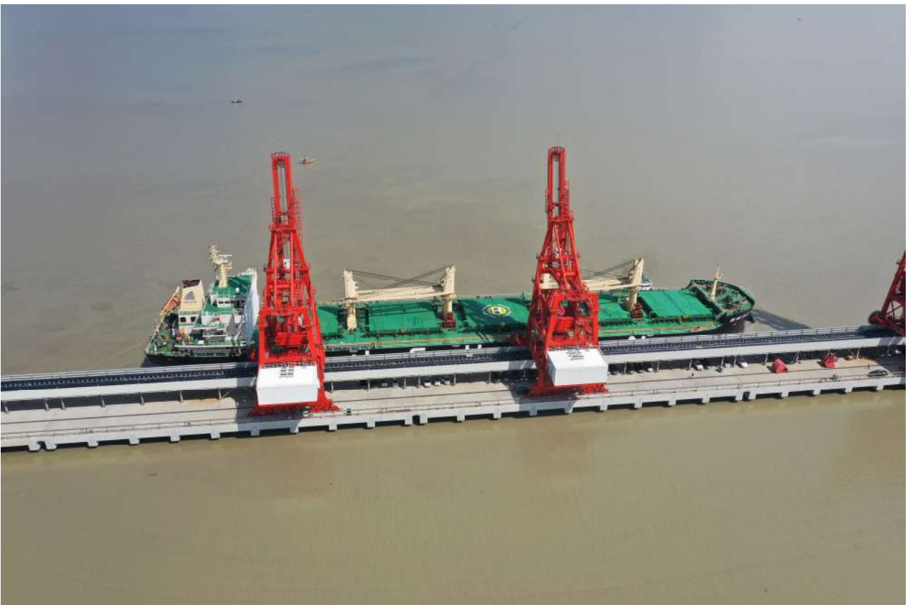
First Coal Laden Ship arrived at Payra 1320 MW Thermal Power Plant (1 st Phase) (Under JVC)
